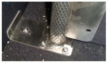
**Step 10** – If the Partition is getting 1 or 2 shelves, pre-attach the appropriate number of angle brackets (2 for each shelf) to the lower partition wall. The Brackets must be attached to the face opposite the tongue side of the partition as shown.
